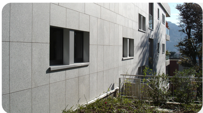
Cantiere Indra - Lugano - granito sardo Indra construction site - sardinian granite
